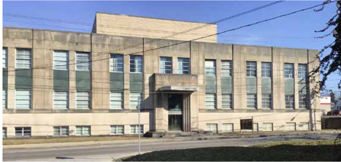
Shelby Mutual Insurance 1953 building at 19 Mansfield Avenue. Photo courtesy of City of Shelby.
