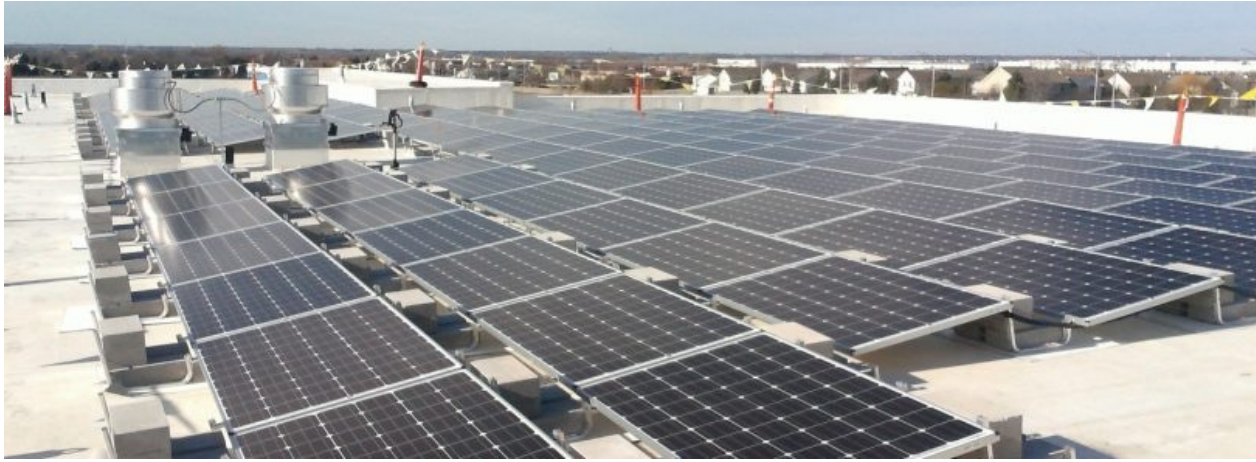
Flat roof parapet installation at Joliet Junior College. Photo: IMEG Corp.
