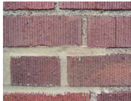
Recent poor repointing. New mortar has been smeared onto the face of the brick and does not match original mortar in color, texture or tooling.
