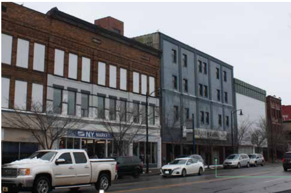
An example of unsuccessful solid/void patterning in newer construction.
