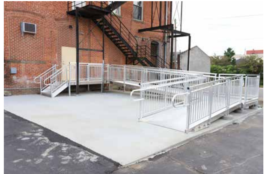
The rear entry to this historic building has added this ramp and parking space for accessibility to the main areas of the building.
