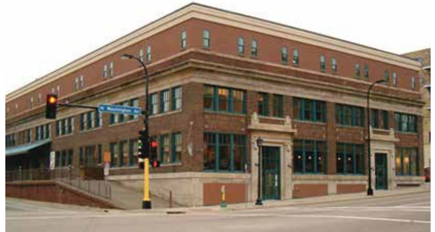
Example of a poorly designed roof addition to an existing structure
