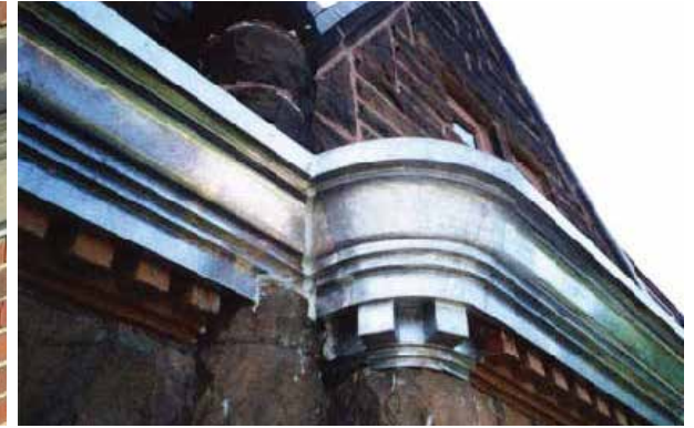
Missing elements are replaced with material to match and look like the original.
