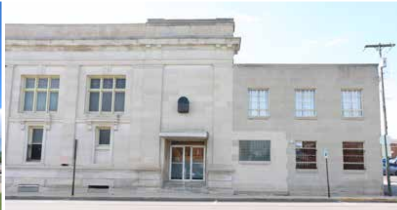
This historic bank has a rear addition for extra office space. The addition respects the historic building in scale and its proportion of openings, and the style and character of a more modern design.
