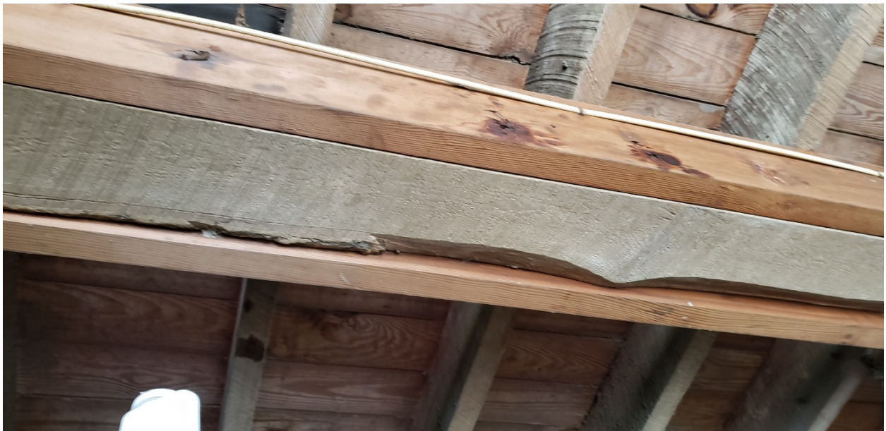
Construction inside the barn indicates roughly sawn lumber and rough-cut beams, suggesting it was possibly built in the mid- to late-1800s.
