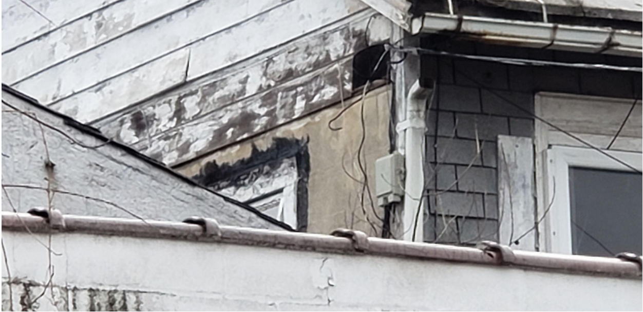
Stucco is still exposed on the rear wall of the building from a renovation in 1924.
