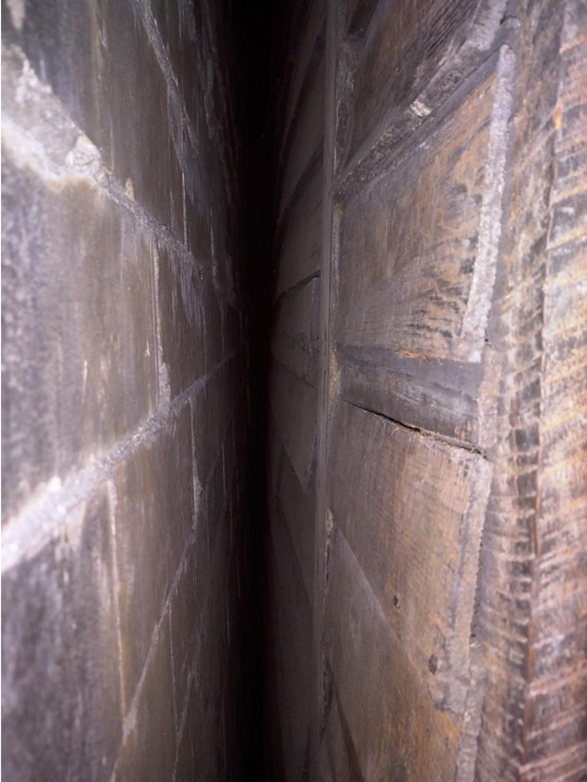
Wall between 13 and 15 North Broadway. Original lap siding on 13 Broadway, right, is still visible.
