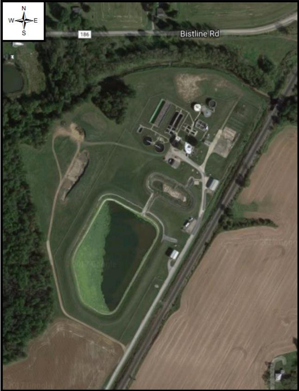
Figure 2: Shelby Wastewater Treatment Plant
